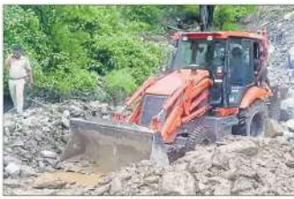
Machines deployed to clear the Mandi-Kullu NH which was blocked due to heavy landslide near Pandoh on Saturday. PHOTO
